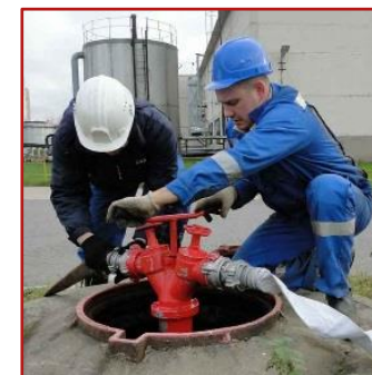
emergency water supply
