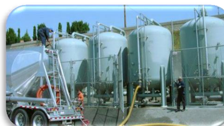
Natural gas storage
